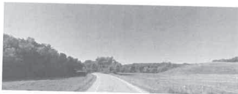
Shaw Road looking south toward Fawn Creek Crossing.
