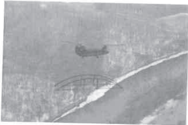
Photo 1 shows a Chinook Helicopter moving the bridge from Hale to the park. Photo 2 shows the bridge as it stands today.
